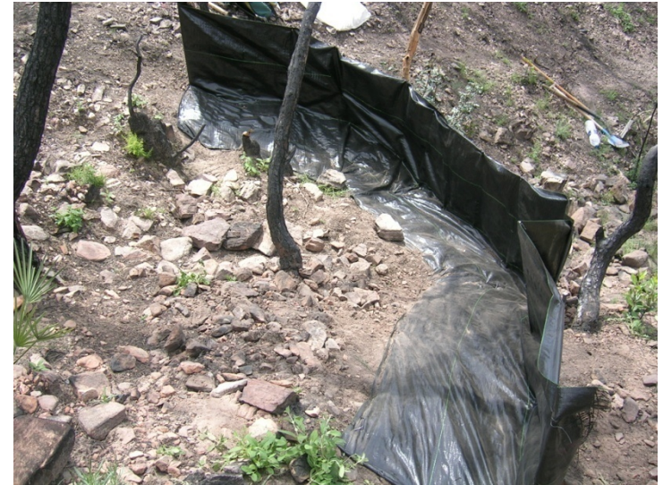
Silt-fence used to monitor sediment yield
