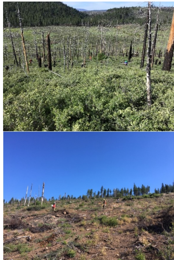
Figure 2. Pre (a), and post (b) site preparation. Pre-treatment (a): extensive, continuous shrub cover with many standing dead trees characterize the area. Post-treatment (b): shrub cover is limited to small, scattered patches with shorter stature. Few snags remain but a scattering of fine fuels is visible. Areas in (a) and (b) are representative but are not identical locations.
