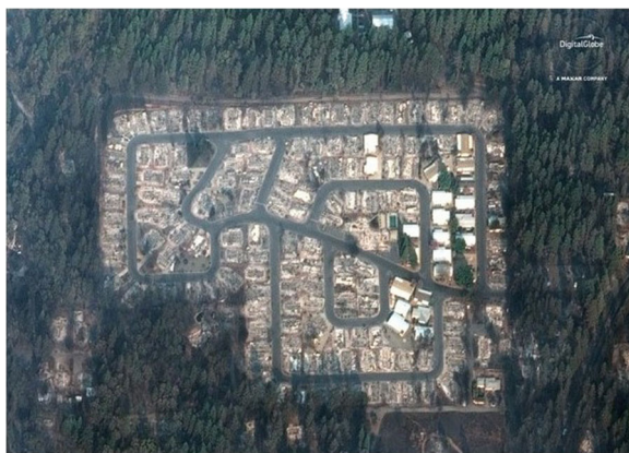
Fig. 7 The Kilcrease Circle community in Paradise, California, USA, devastated by the Camp Fire, surrounded by green forest with canopies largely untouched by fire. (DigitalGlobe, a Maxar company satellite image from Nov 2018, used by permission; https://digitalglobe.app.box.com/s/um3og59f92yx0sit0c07p7gremd7r1vj )
