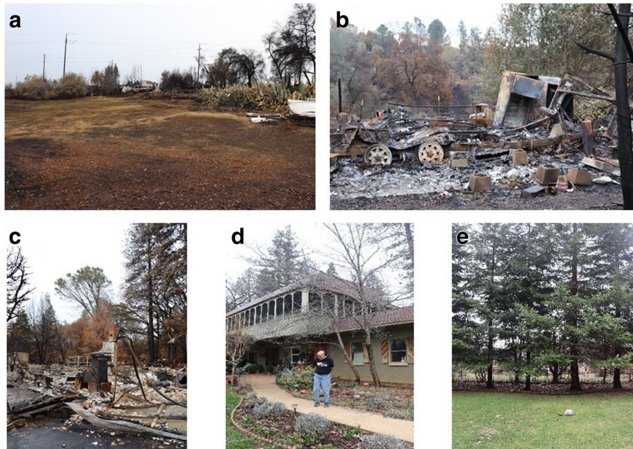
Fig. 6 (a) Home incinerated with very little vegetation surrounding the home, illustrating the role of embers, not radiant heat of the fire front (actually, lack of vegetation may have contributed to more rapid laminar flow of the ember load to the house). (b, c) Homes incinerated while adjacent green trees survived. (d) Home unburned while homes within 30 m were destroyed. (e) Home that survived had a border of green trees between it and adjacent destroyed homes, perhaps acting as a barrier to embers hitting the house. Photo credit: Jon Keeley, USGS, Nov 2018, in the town of Paradise
