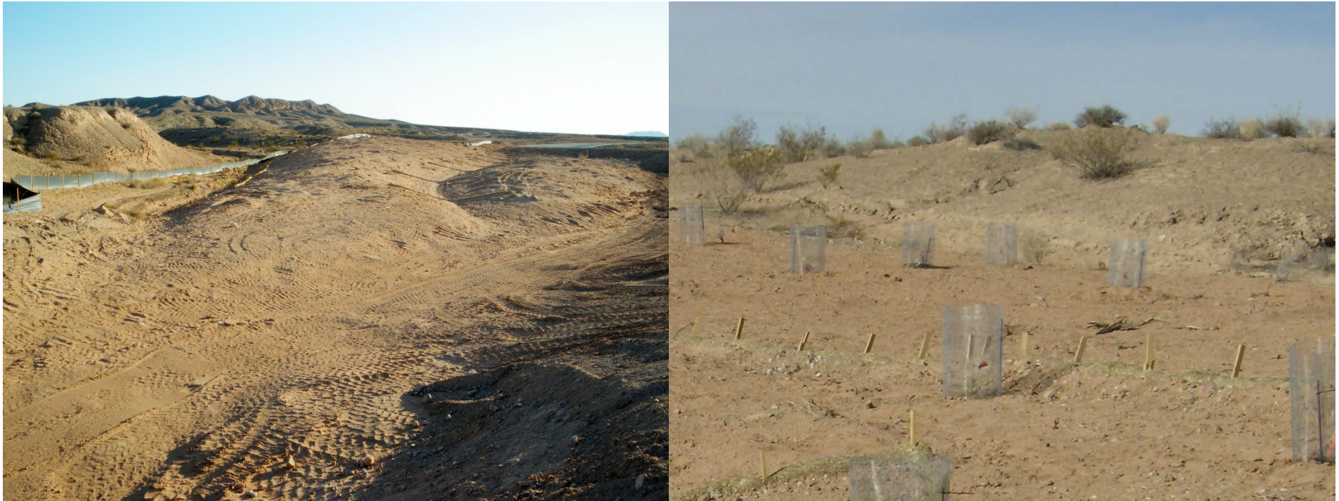
Fig. S3. Images from the Northshore Road realignment project in gypsiferous soils, in the eastern Mojave Desert, USA. (Left) Northshore Road realignment 14 months (December 2009) after construction was completed and salvaged topsoil reapplied to newly contoured surfaces. In the image, topsoil is restricted to the main contoured areas and is not present in the constructed dry wash area. Washes were not included in the study. Surface material was reinforced by straw barriers. (Right) Image of the Northshore Road revegetation project established 15 months after construction disturbance began and one month after topsoil was reapplied to study areas. Planting treatments were assessed in Abella et al. (2015). Ambrosia dumosa shrubs from this project were used as a treatment in our biocrust restoration study. Photographs by L. P. Chiquoine.
